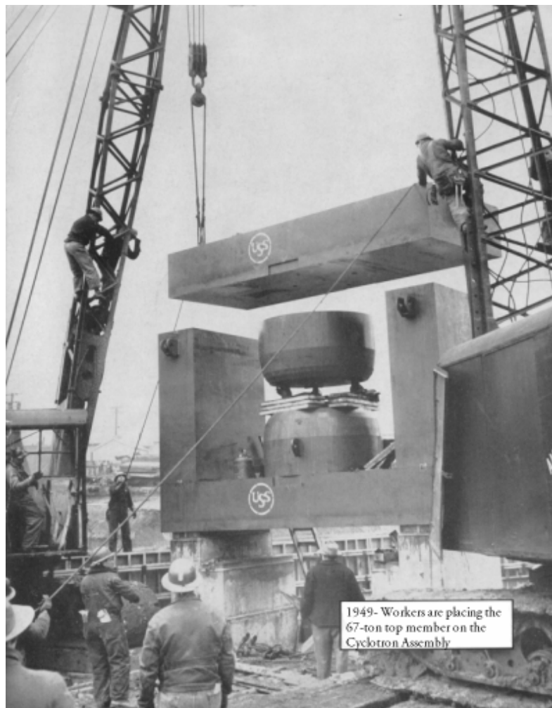
Figure 2 – 1949 Construction Photograph of Cyclotron Electromagnet.
