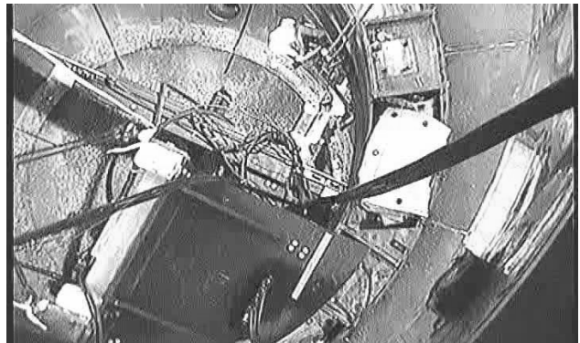
Figure 7, Bridge view of 38i after lower head cuts
