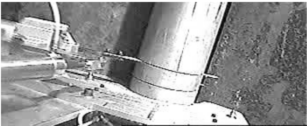
Figure 11, Pipe Saw cutting MT outlet pipe
