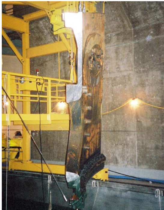
Fig. 3. Core support shield segment.
