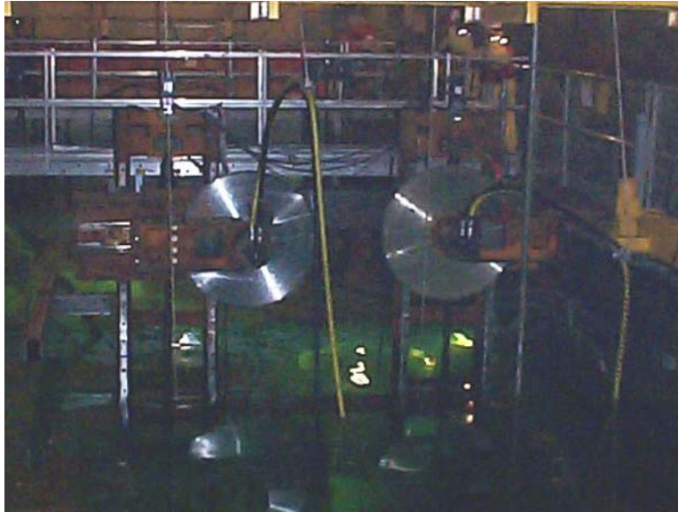
Fig. 4. 38i II installed in cavity.
